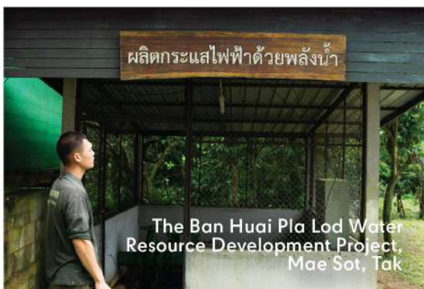
The Ban Huai Pla Lod Water Resource Development Project, Mae Sot, Tak
